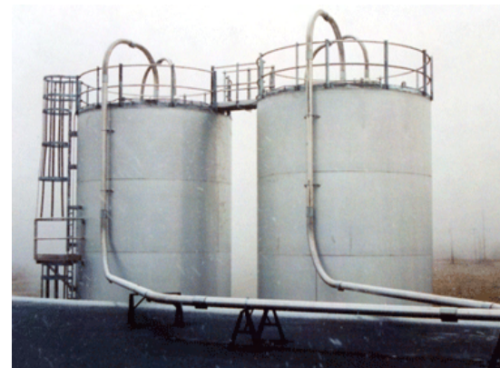
Tank & vessel construction
