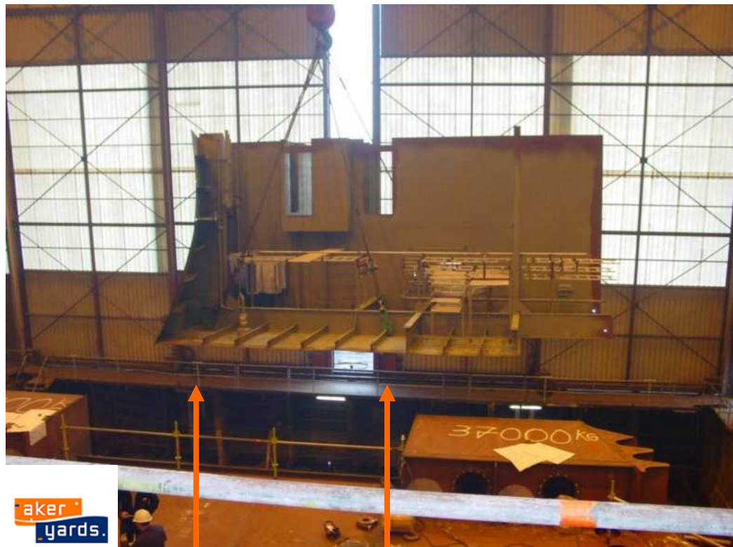
Transport of ship section by using IPSBUSUZ lifting clamps.
